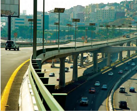
The project is structured in three phases: the first phase comprises a reversible 22-kilometer viaduct between "El Toreo" and "Tepalcapa". The second phase will comprise a parallel viaduct to be built when maximum traffic density along the former has been reached. Finally, a third phase will extend both viaducts by 10 kilometers.
